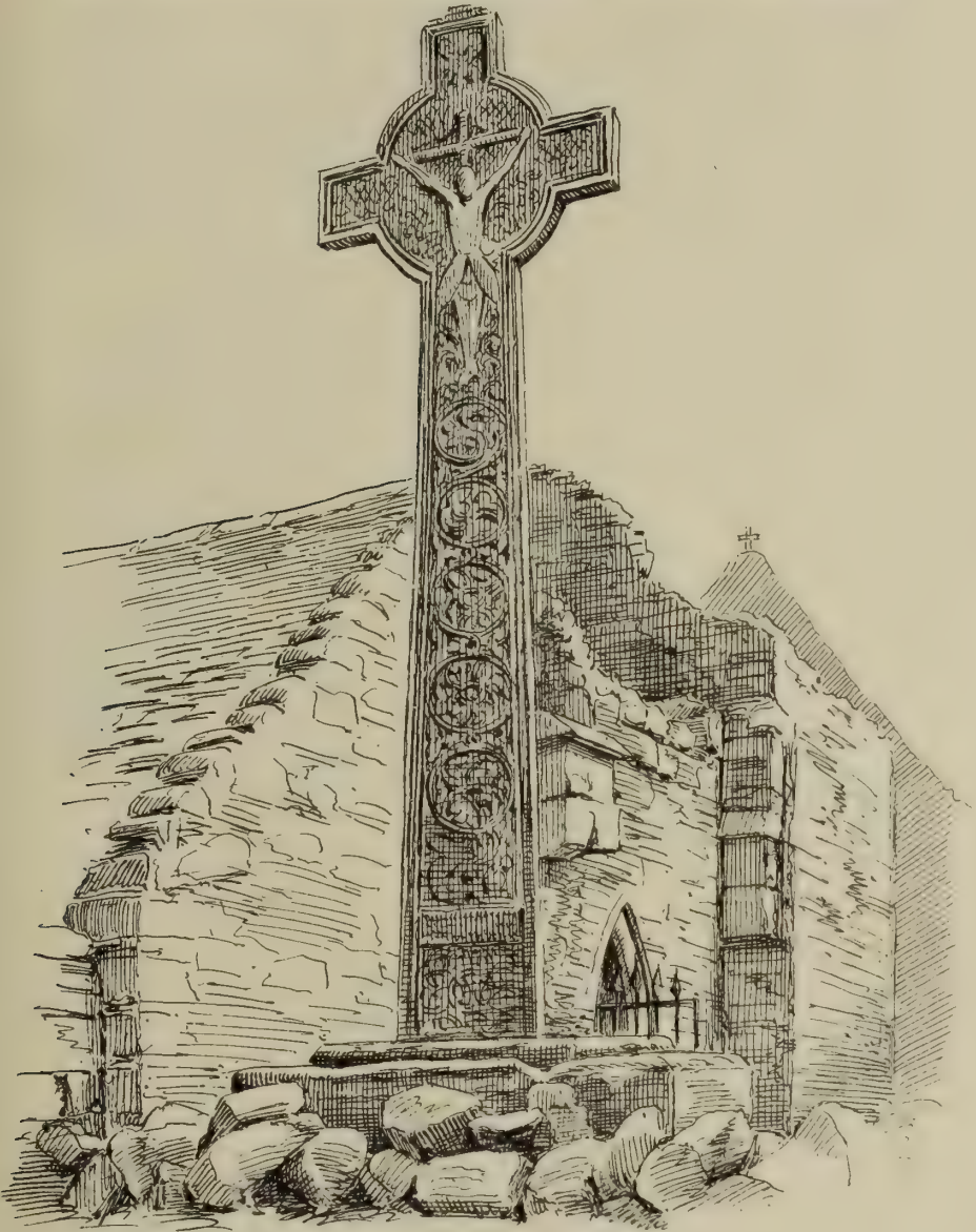
FIG. 1310.—Oronsay Priory. Cross and South Side of Narthex and Church.
